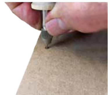
Drill or punch the holes
