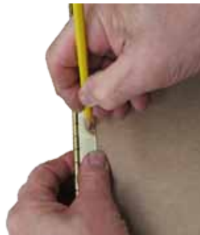
Hold the hinge tight, trace the holes
