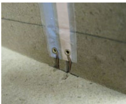
... wired thru drilled holes in the Base Floor
