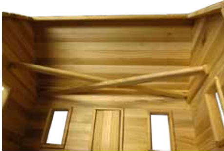
Loft Logs: temporary bracing
