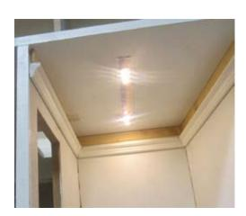
Test - if it doesn't light, you may have to switch the wires at the transformer (to make the copper the "+" leg of the wire.
