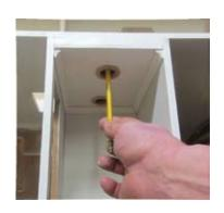
Trace the opening onto the structural ceiling.
