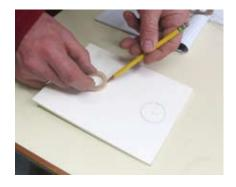
Trace the narrow ring of the Frame onto the False Ceiling.
