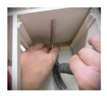
Eyelet the Tapewire to the Ceiling Run, copper-to-copper and blue-to-blue.
