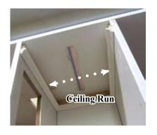
Lay tapewire that extends past the tracings and overlaps the Ceiling Run (note: the LED can not be installed where the runs overlap).
