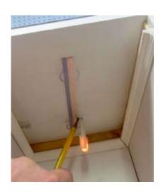
Test and mark the Ceiling Run.
